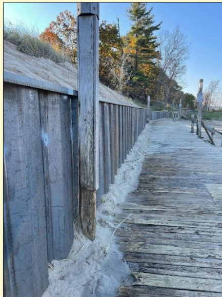
New retaining wall along the south boardwalk
